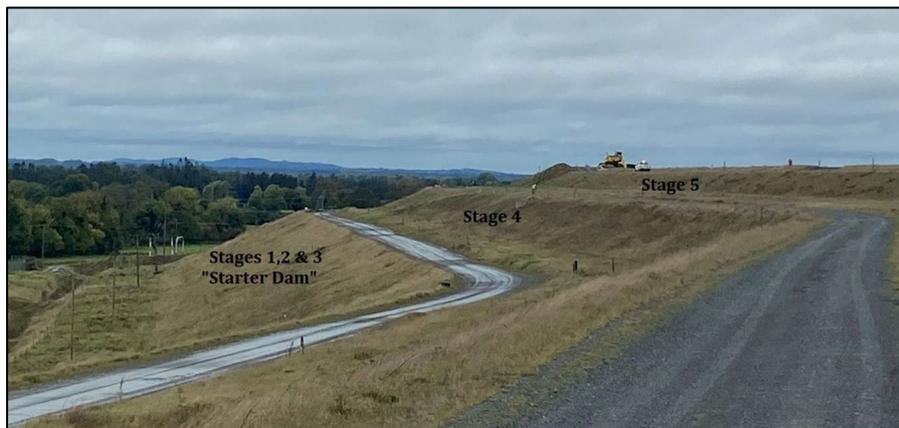
Figure 11. 2: Embankments side profile
